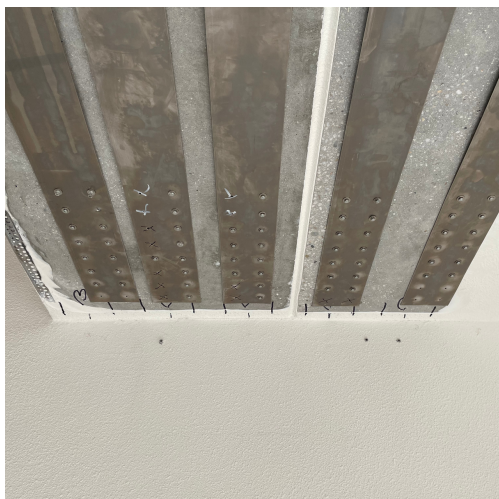
Close up verankeringen re-plate
